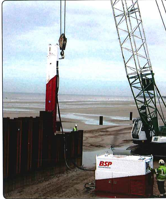
Above: Various SL30 Hammers fitted with legs and inserts for diving sheet piles. All are shown in crane suspended operation and powered by BSP Power Packs.
